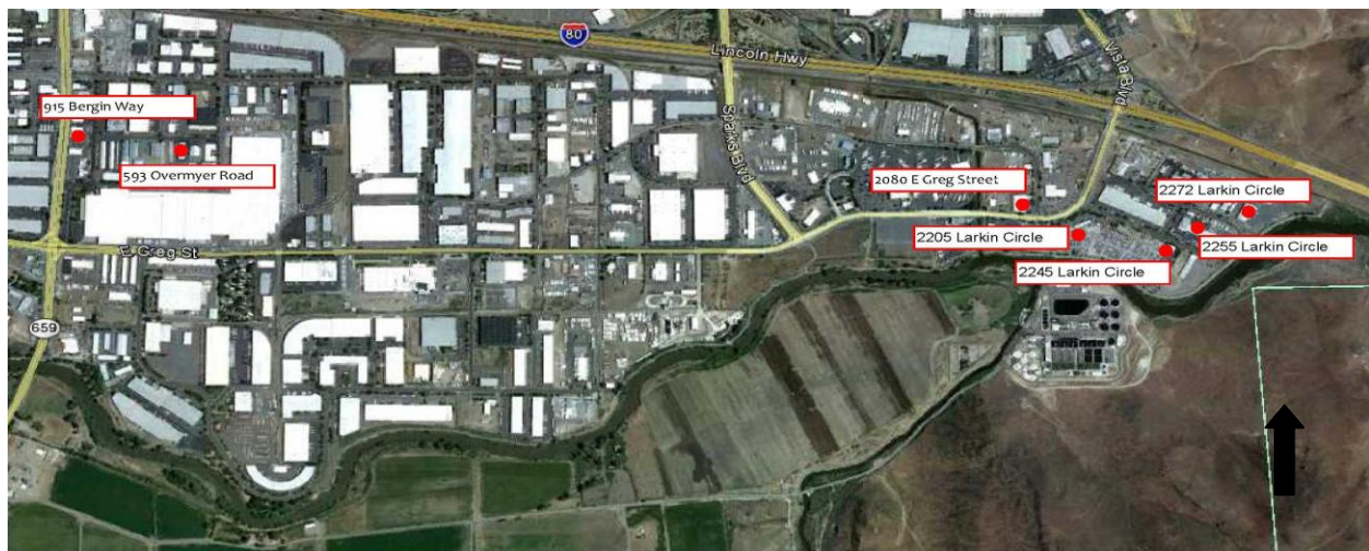
Figure 1: Aerial view of the 7 non-compliant structures identified during previous 2009 CAV
